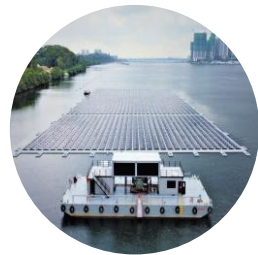
Floating Solar (FPV)
